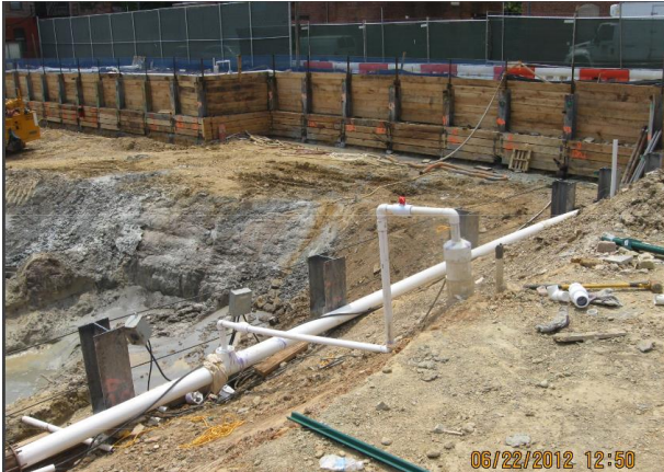
^Pictured above is the actual excavation of the southern building foundation, compliments of Balfour Beatty Construction.
